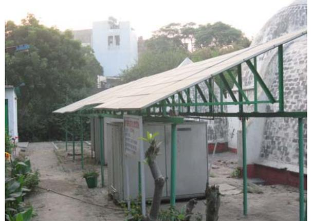
**Figure 2. A 2.32 kW<sub>p</sub> Stand-alone PV system**
