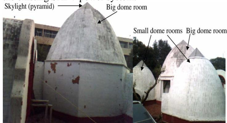
**Figure 3. Skylight integrated with the Mudhouse**
