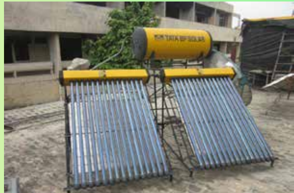
Evacuated Tube Solar Water Collector
